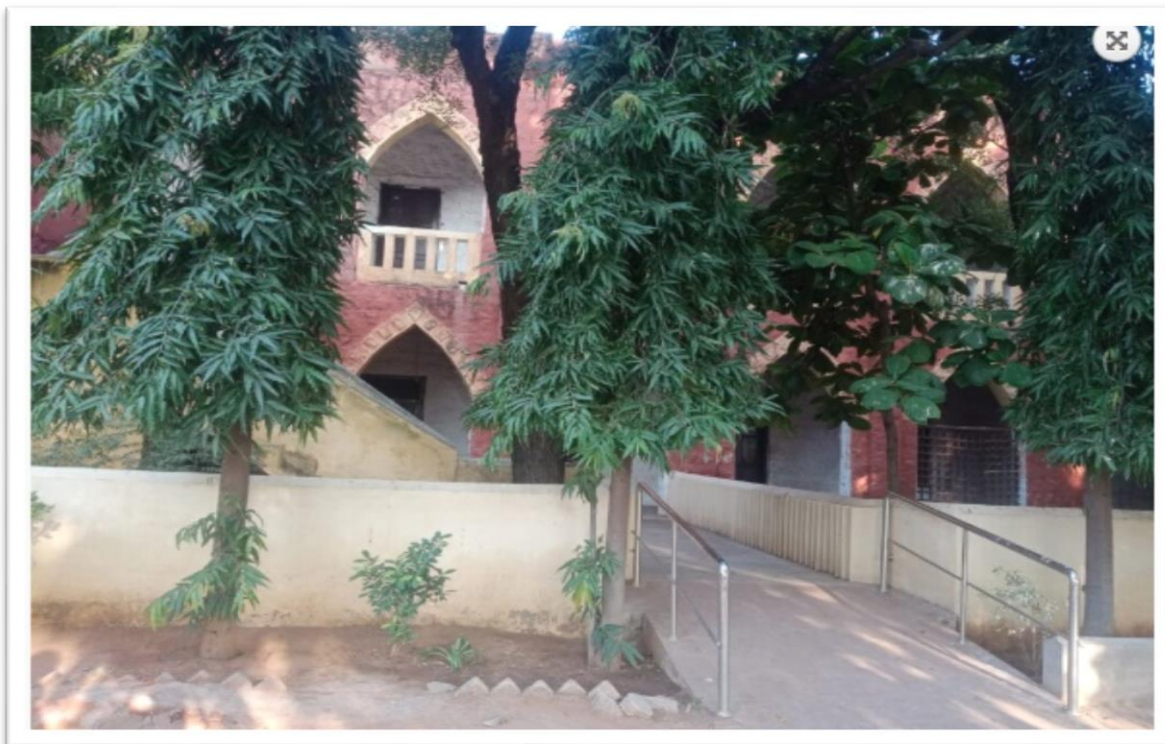
Ramp for Differently Abled in Main Block
