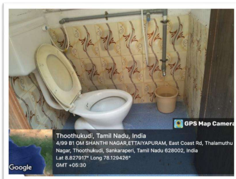
Disabled friendly washroom
