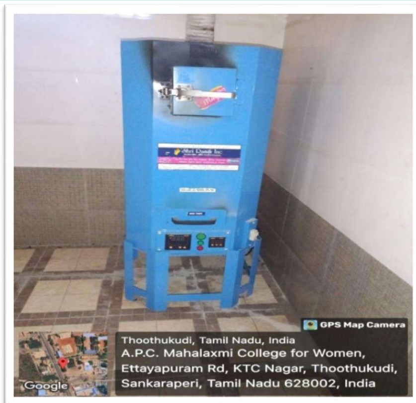
Incinerator at maths block
